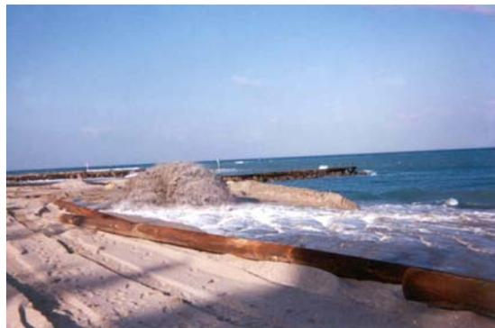
An alternative to the fixed sand bypassing plant is a fluidizer system. This system takes fluidized sand from the ocean or, alternately, from the inlet, and pumps it through pipes to the south beach as fill. The feasibility of this system, as applied to the Jupiter Inlet, awaits continuing experiments currently being conducted at Oceanside Harbor, California, by the Corps of Engineers.
