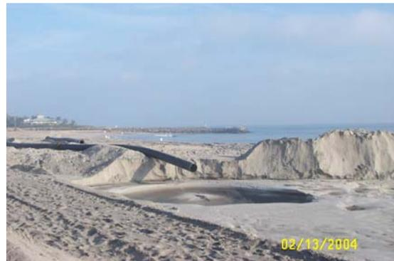
from the trap. To minimize the erosion problem occurring south of the south jetty, the University has recommended that a minimum of 60,000 cubic yards be pumped to the south beach on an average annual basis.
